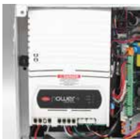
Built-in variable frequency drive.
